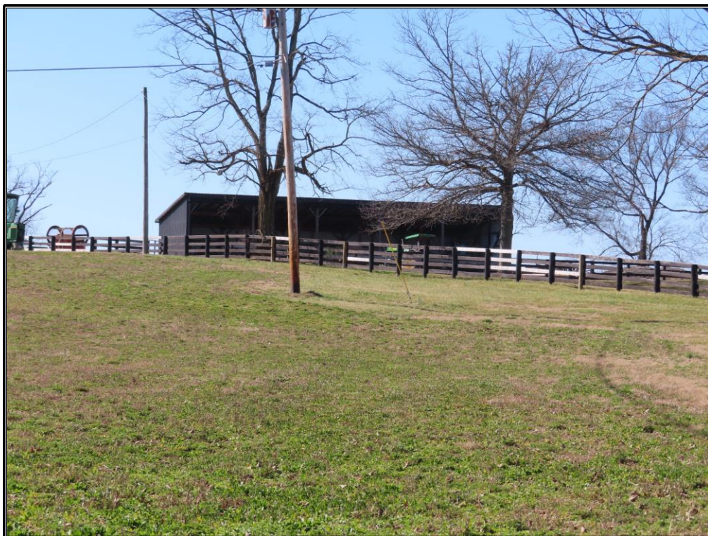
Figure A-8. FR 115. Northeast and southeast elevations of the equipment shed associated with FR 115, looking west.
