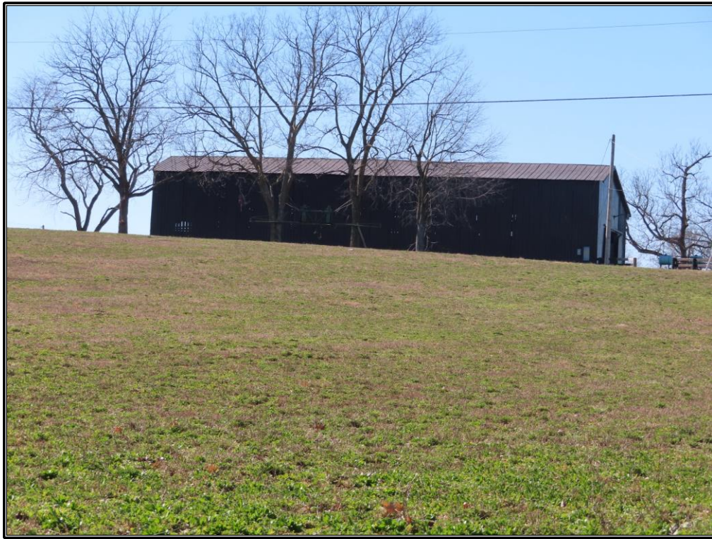
Figure A-9. FR 115. North and east elevations of the first barn associated with FR 115, looking west.
