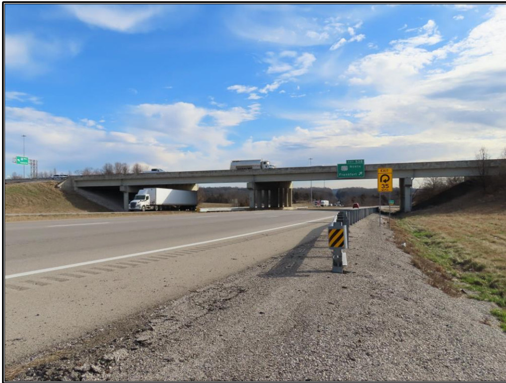
Figure A-1. Overview of the APE from I-64, slightly west of its intersection with the US 127 bridge, looking east.
