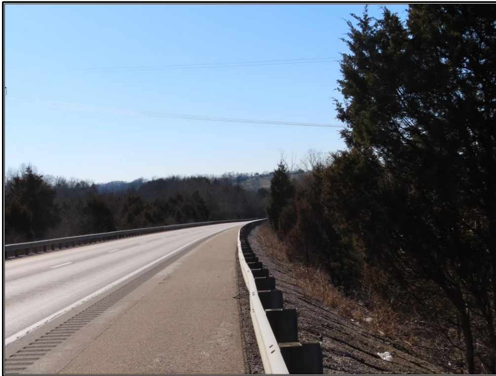
Figure A-3. Overview of the APE from I-64, slightly east of where it spans the Kentucky River, looking west-southwest.
