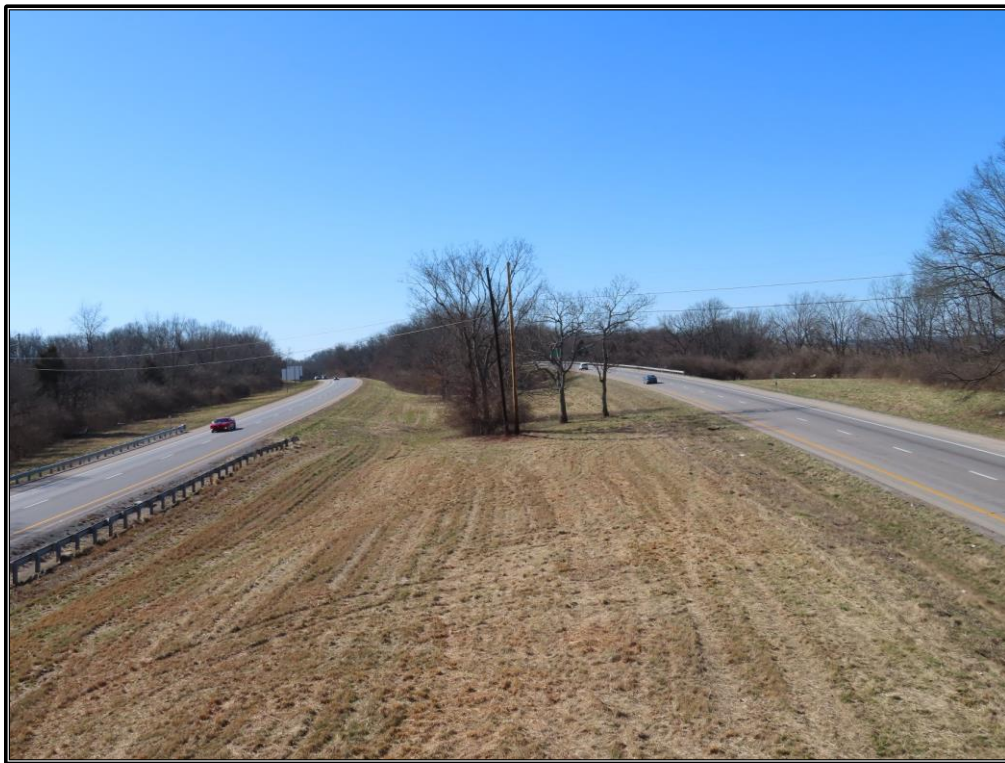
Figure A-5. Overview of the APE from the bridge that carries Hanley Lane over I-64, looking west.
