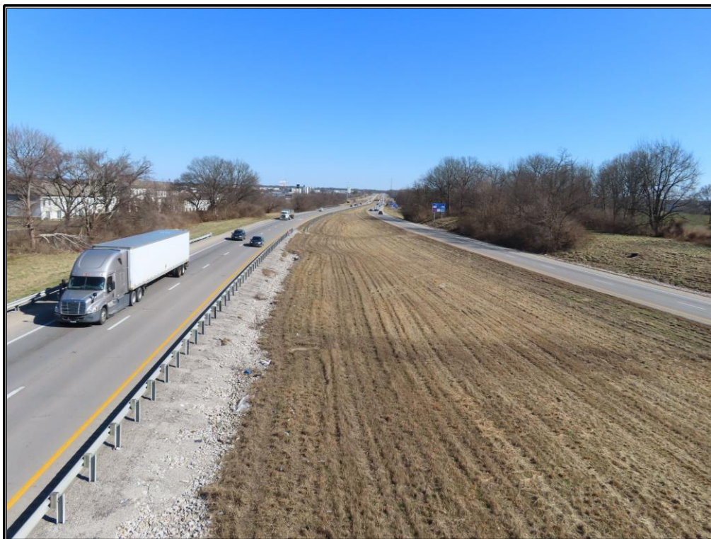
Figure A-4. Overview of the APE from the bridge that carries Hanley Lane over I-64, looking east.
