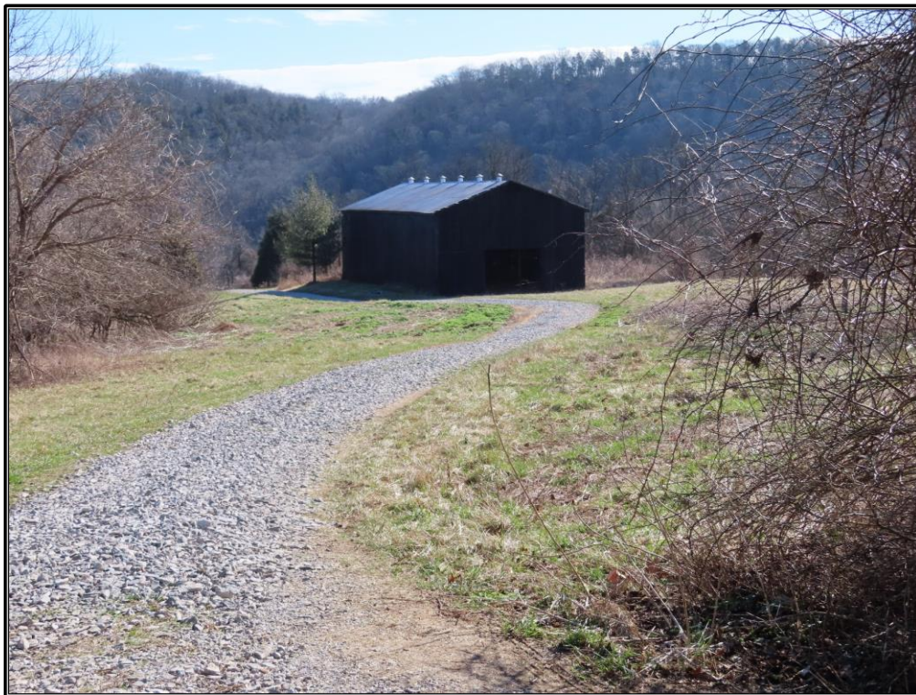
Figure A-11. CRA 1. North and west elevations of the barn, looking southeast.
