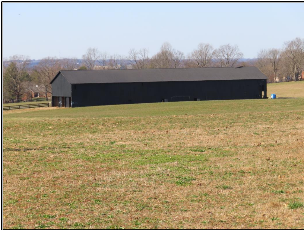
Figure A-10. FR 115. Southwest and southeast elevations of second barn associated with FR 115, looking northwest.
